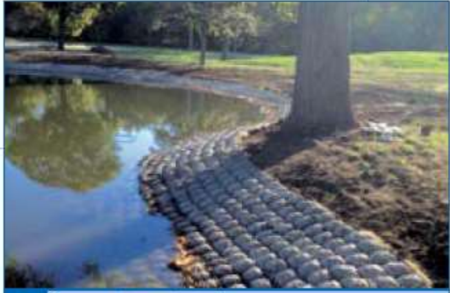
7 Sycamore tree protected.
