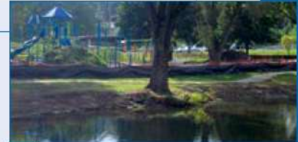
1 Sycamore tree erosion.
